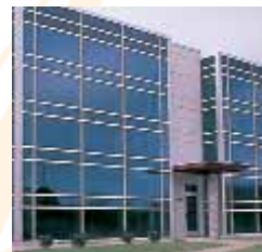
The new 50,000 square foot Shell Industrial Building is open for business.
